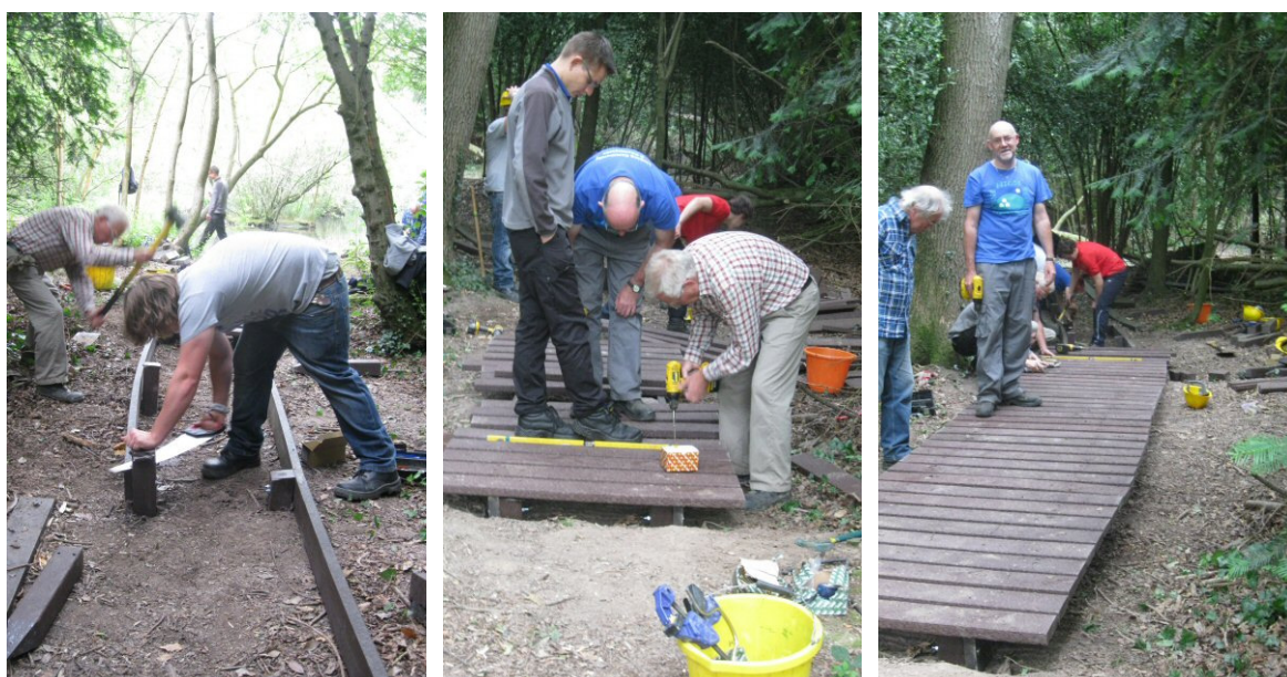
Volunteers are building a new boardwalk on Lamberhurst Common from recycled plastic materials.
